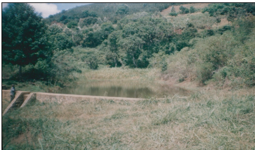
Photo 5.2: An Improved Ndiwa Structure at Shashui Village
