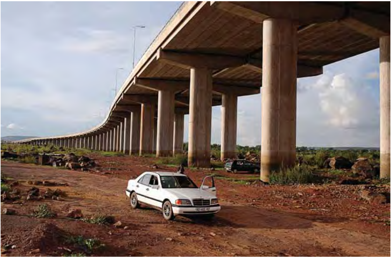
A bridge built in 2011 by China Gezhouba Corporation in Mali's capital city, Bamako.
