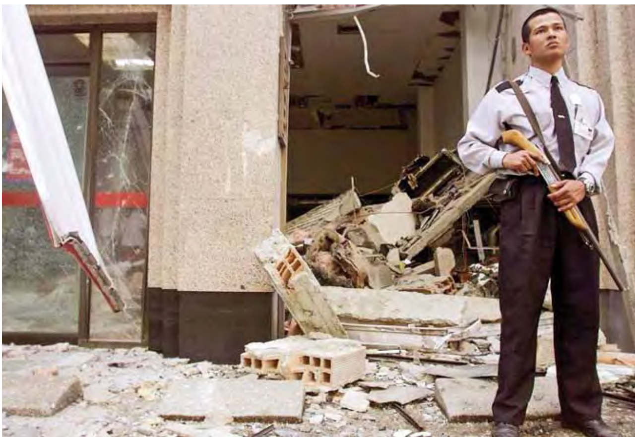
A member of a private security company stands guard next to the remains of a bomb-damaged bank in Medellín, Antioquia province, Colombia. The attack was made by Revolutionary Armed Forces of Colombia (October 2002).
