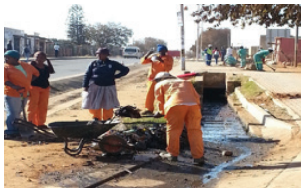
Photo 3: The CWP in Ivory Park clearing rubble and dirt from the stormwater drainage system.
