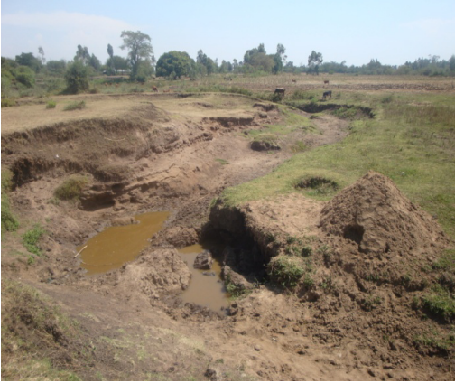
Effects of flooding in Oyola village
