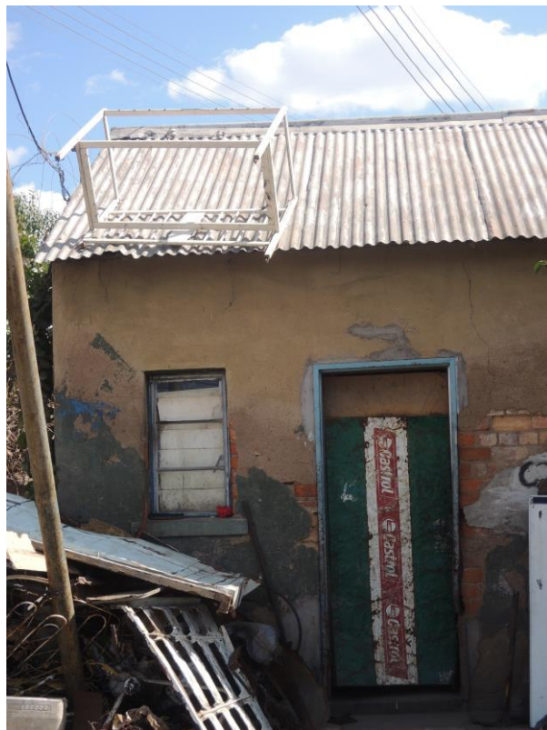
Figure 8: Miners houses in Hwange villages
