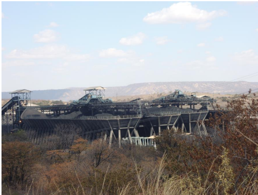
Figure 2: Hwange Colliery Company processing plant
