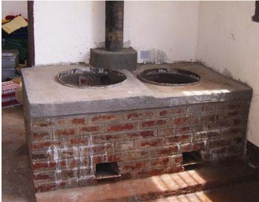
Figure 10: More efficient and healthier use of fuel wood (burnt brick-type, fixed, indoor/outdoor); Source: Wiskerke, (2009; 117)
