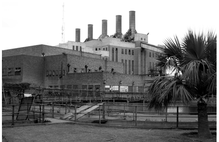
In Zimbabwe, Lahmeyer investigates, among others, the thermal power plant Bulawayo.
