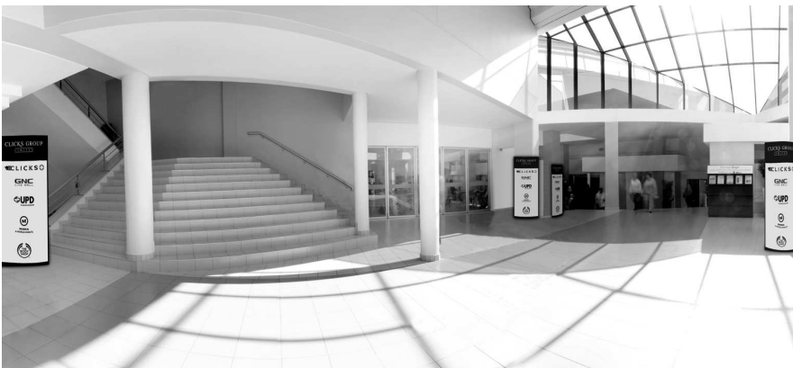
Clicks Group Head Office Building, top ranking building in the National Energy Barometer Survey for the 2012 utility year in the head offices category
