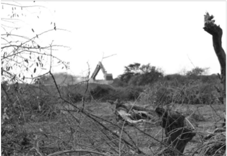
Figure 2: Bulldozer clearing bush along the Lower Omo
