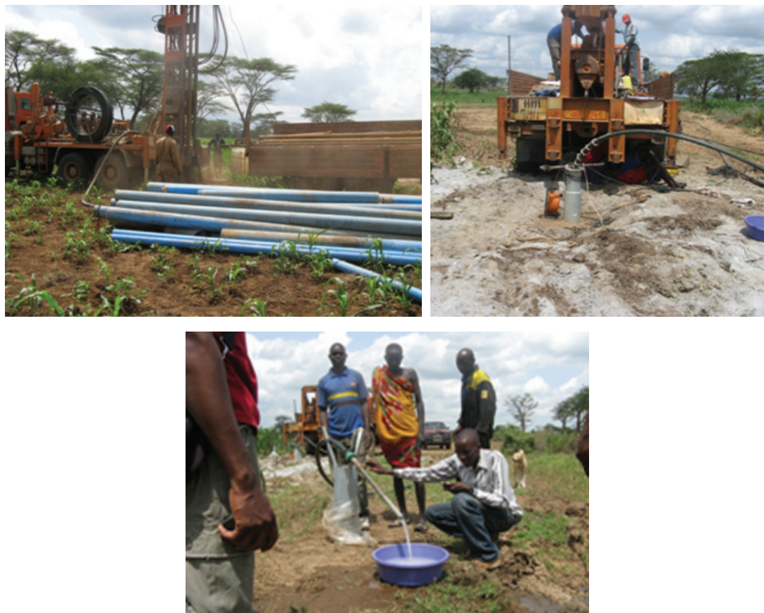
Figure 11: A borehole being drilled in Longoleyek village in Lorengedwat Sub-county to provide clean and safe water for human consumption sponsored by Welthungerhilfe an international NGO operating in Nakapiripirit District
