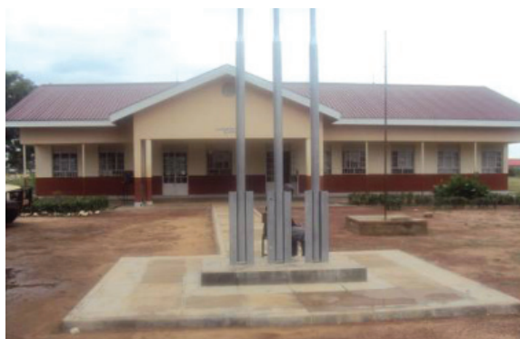
Beautiful administration block of Arengeshiep S.S.S constructed by Irish Aid.
