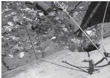
Figure 10 Open sewer drain into Indian Ocean in Lamu (2006)
