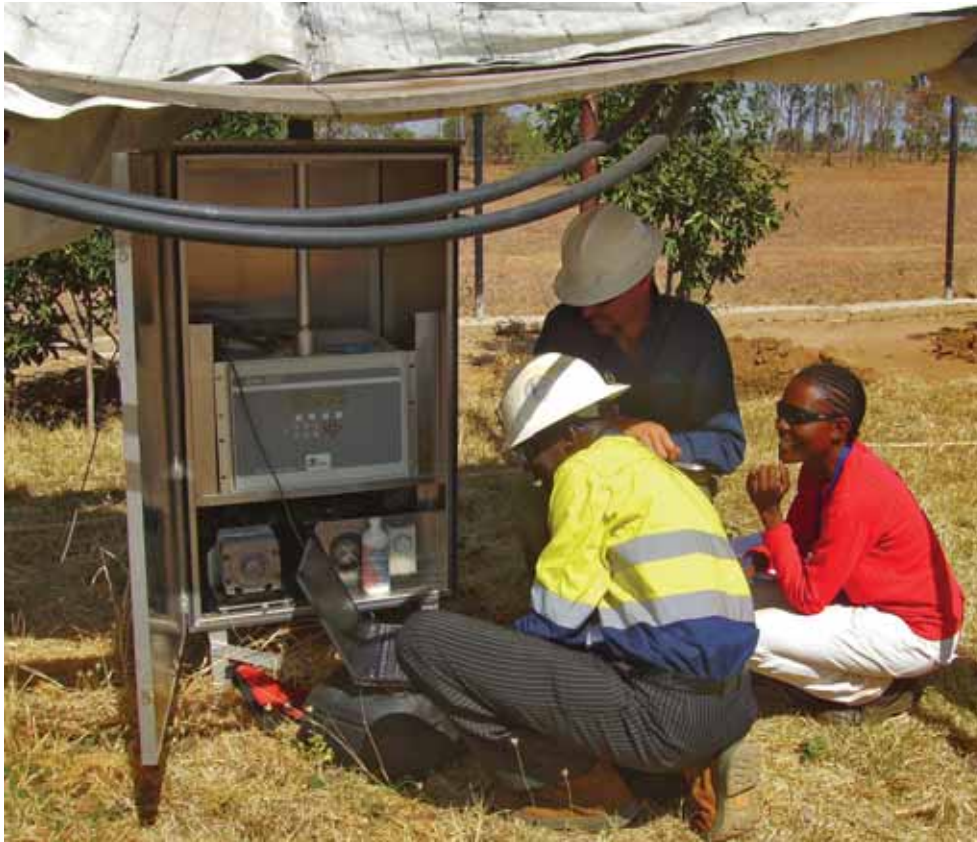
Figure 5: Dust monitoring equipment
