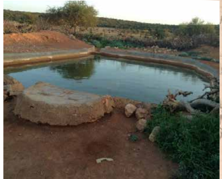
Figure 3 b: Barkad without a cover at Kalabayr due to loss of traditional cover, duur, June 9, 2016.
