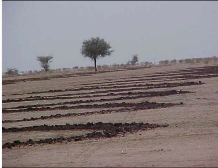
Plate 3. Construction of crescent-shaped terraces (May 2003)
