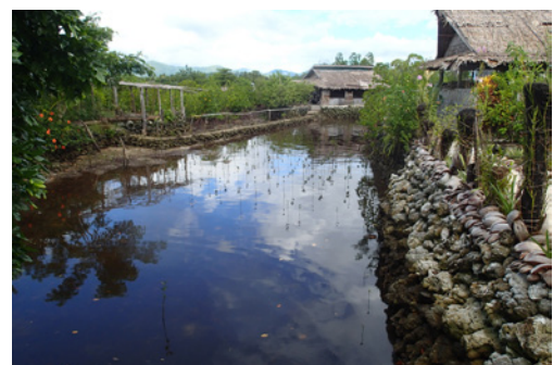
1 3 Image: © World Fish | Hybrid measures: a combination of built 'hard' coastal protection combined with ecosystem-based measures.
