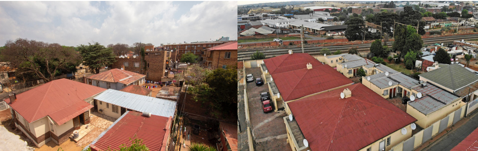
Backyard developments in Yeoville (left) and Malvern (right)
