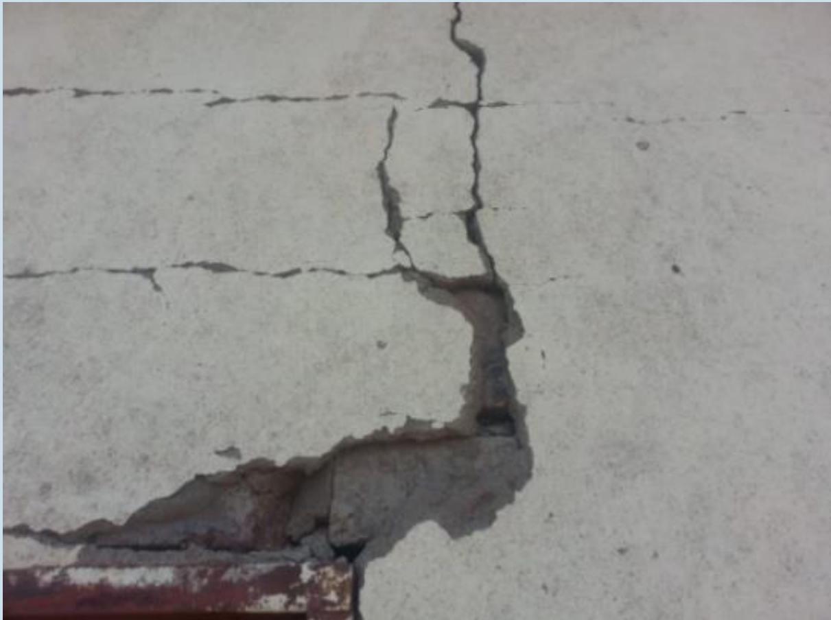
A classroom block at Shonhayi Secondary School cracked due to blasting
