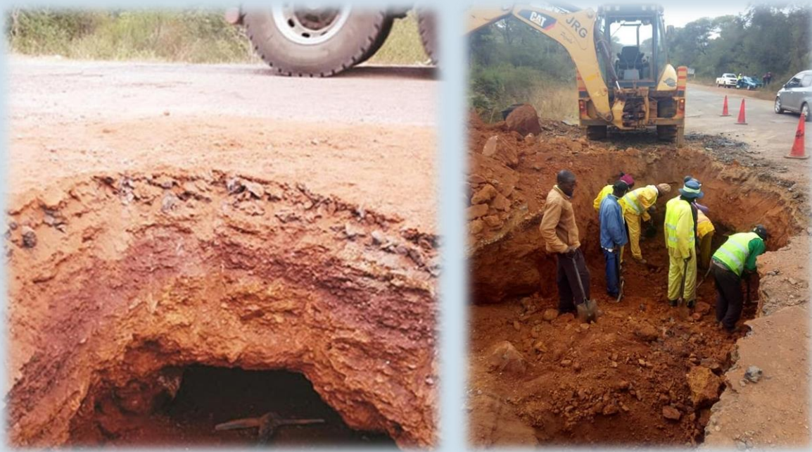
Gweru -Zvishavane, Boterekwa road collapses due to underground illegal mining activities
