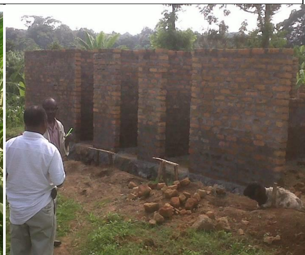
Figure 4.12: A Storage Facility under Construction, Kibosho Area
